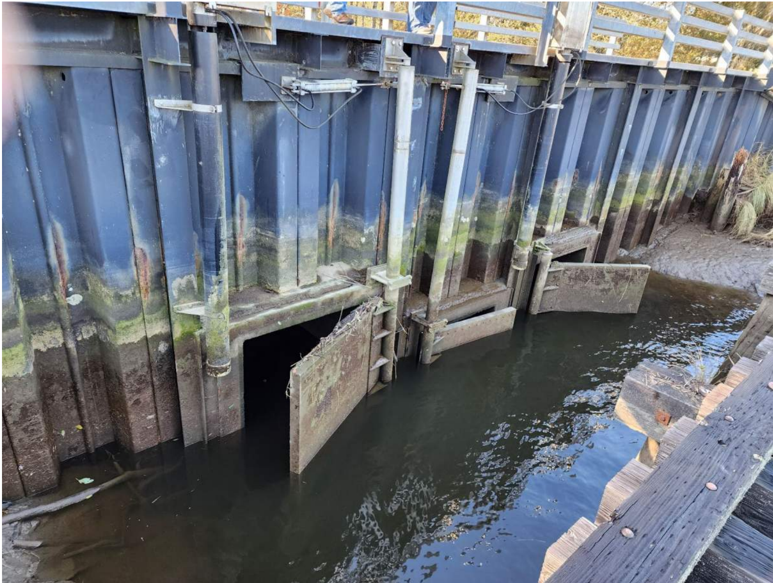
Figure 2. Existing Tide Gates
