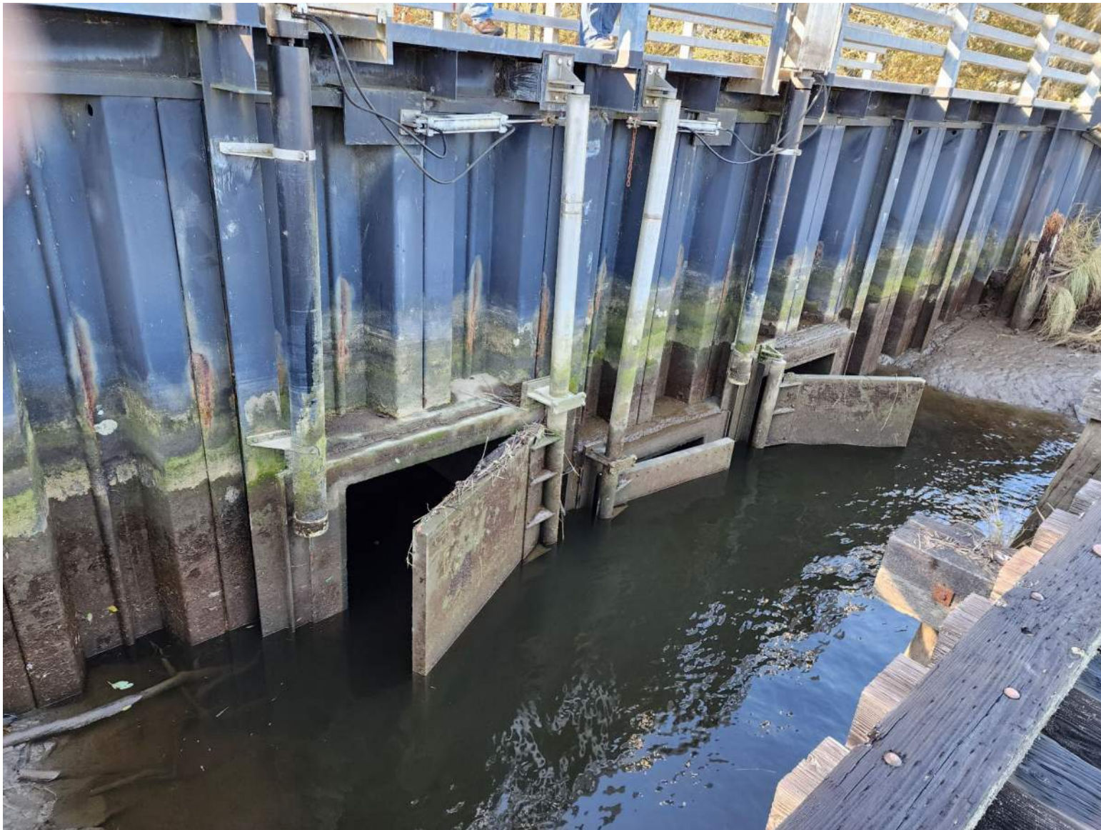
Figure 2. Existing Tide Gates (Downstream side)
