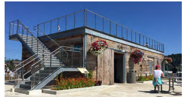
Top: Example of a paved boat ramp | Middle: Example of floating docks for small watercraft access | Lower: Example of a restroom facility with view deck in Gig Harbor, WA (Source: Stantec)
